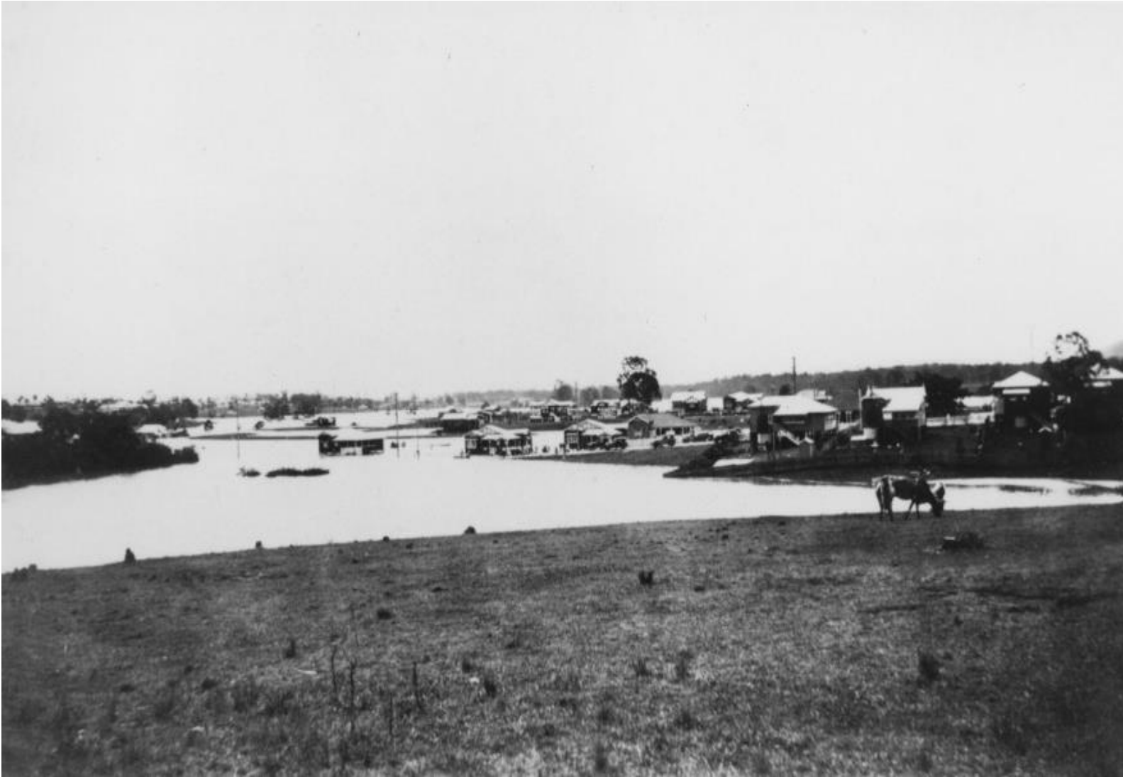
Looking down at Fairfield from Dutton Park, 1930
