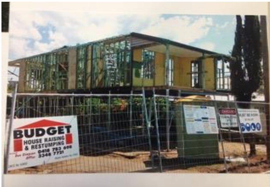
View from Soden Street during renovation
