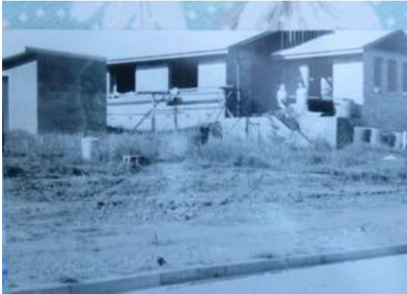
John Ehm's house, 22 Lisle Street under construction. Photo Alex Romow
