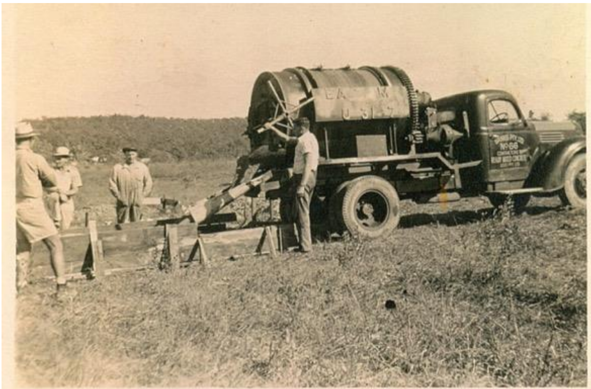
Ready-mixed concrete delivery for John Ehm (in the overalls), 22 Lisle Street c1954. Photo David Baddiley
